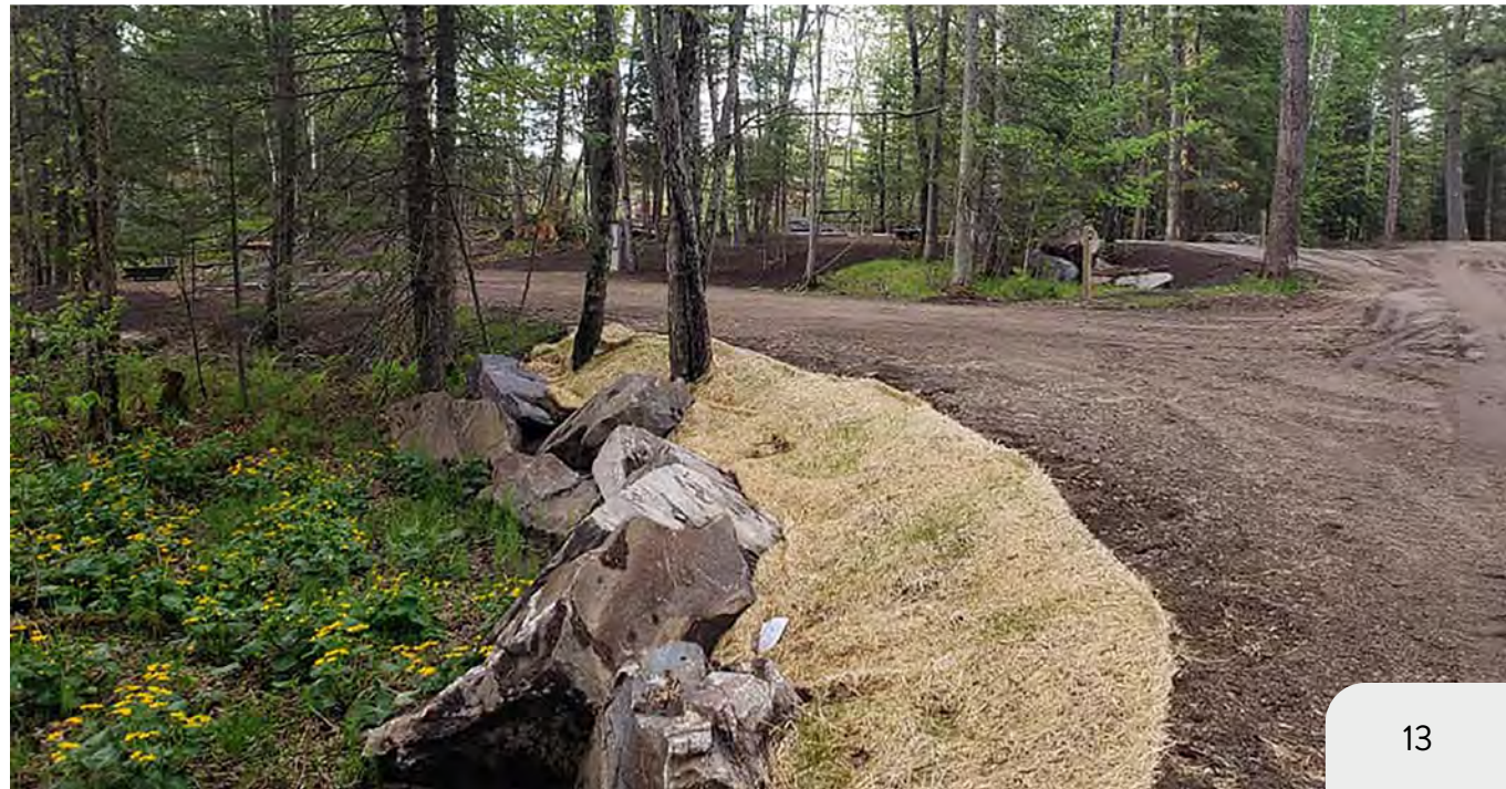
Big Falls Campground and Horse Camp
