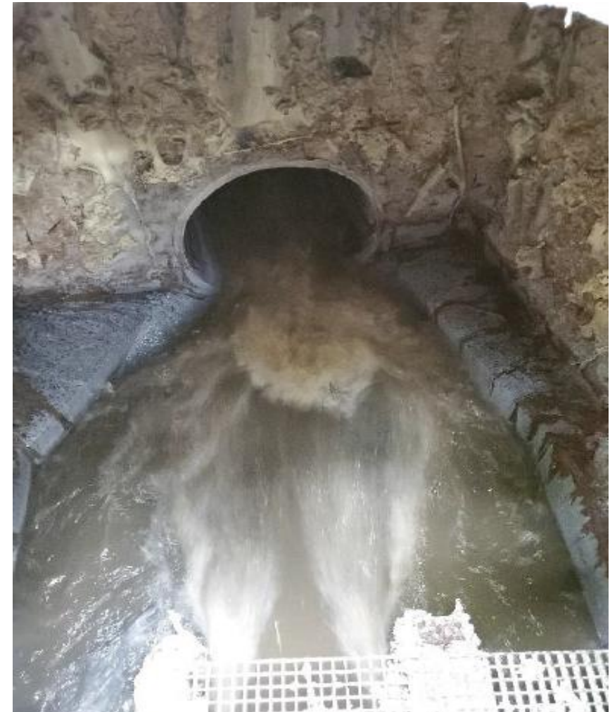
Discharge Maintenance Holes
