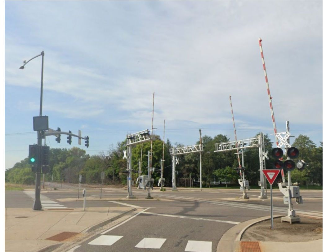
63 rd Ave and BNSF crossing
