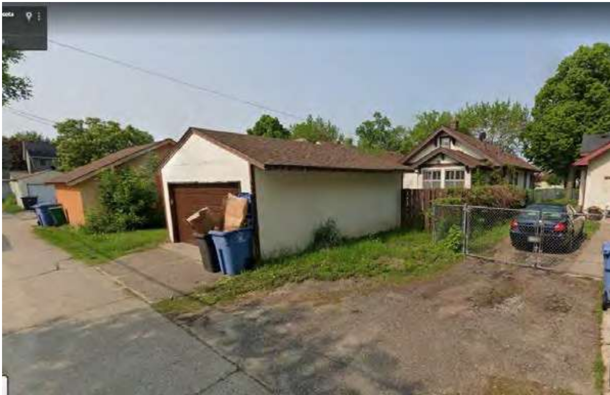
HE-MPC-9170, May 2019, rear elevation and garage, view west (Google Street View image).
