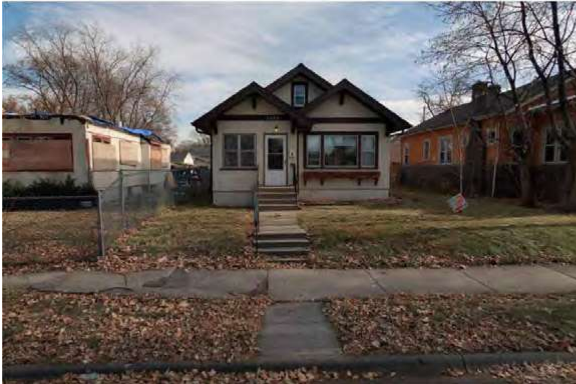
HE-MPC-9170, November 2020, front elevation, view east (Hennepin County Cyclomedia image).
