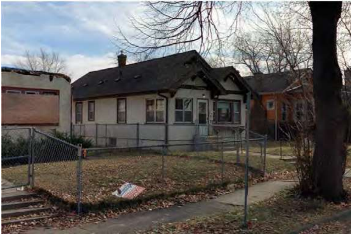
HE-MPC-9170, November 2020, front and side elevation, view southeast (Hennepin County Cyclomedia image).
