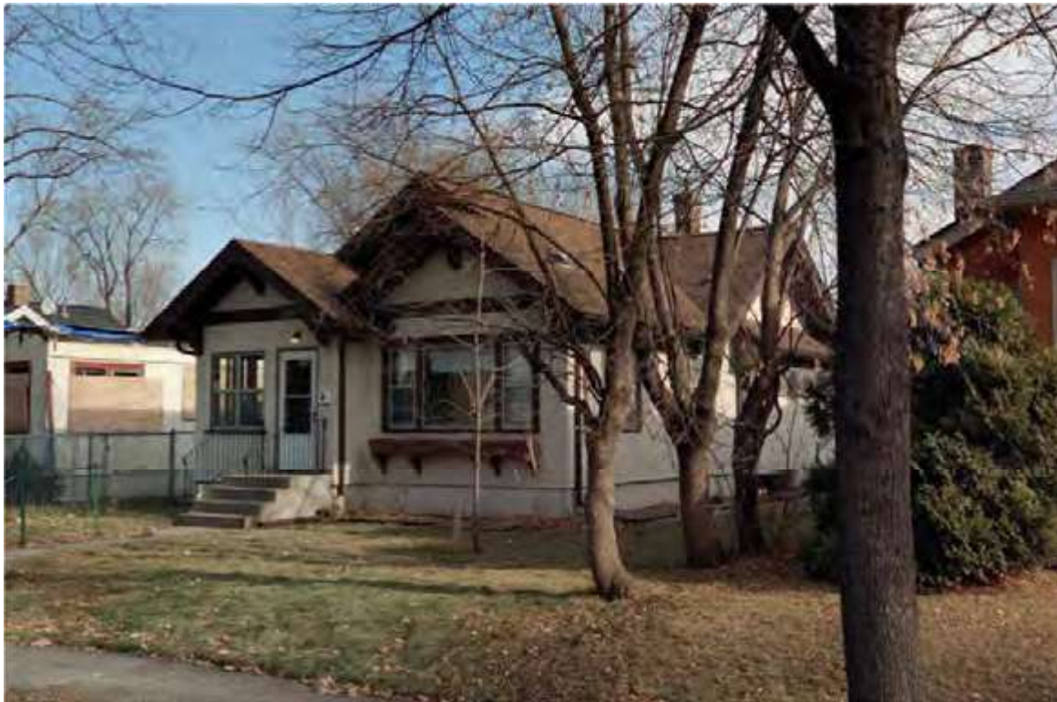
HE-MPC-9170, November 2022, front elevation, view northeast (Hennepin County Cylcomedia image).
