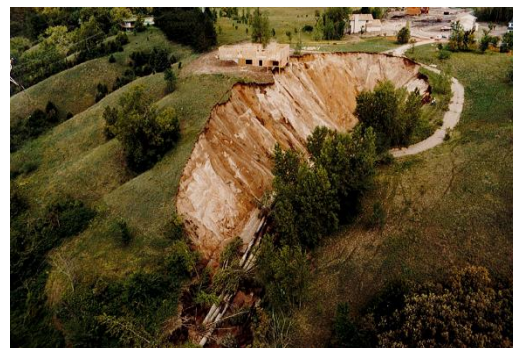
Figure 2: Interceptor failure - Minnesota River
