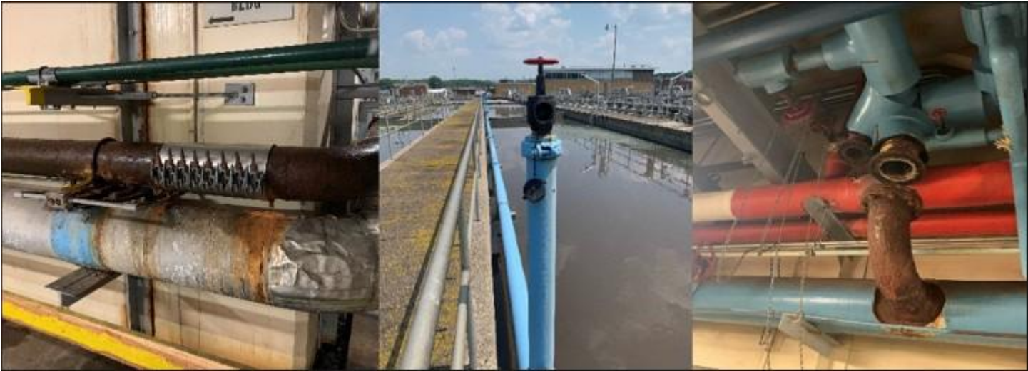
Left: Deteriorated service water piping to be renewed/replaced. Center: Aeration tank spray water piping to be repurposed. Right: Abandoned/obsolete process piping to be removed.
