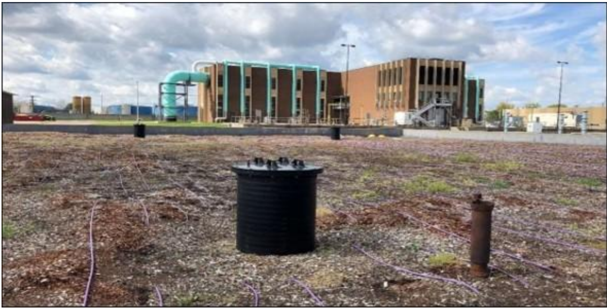
Existing East Pretreatment Biofilter
