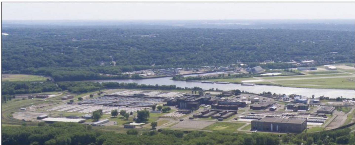
Metropolitan Water Resource Recovery Facility (WRRF)
