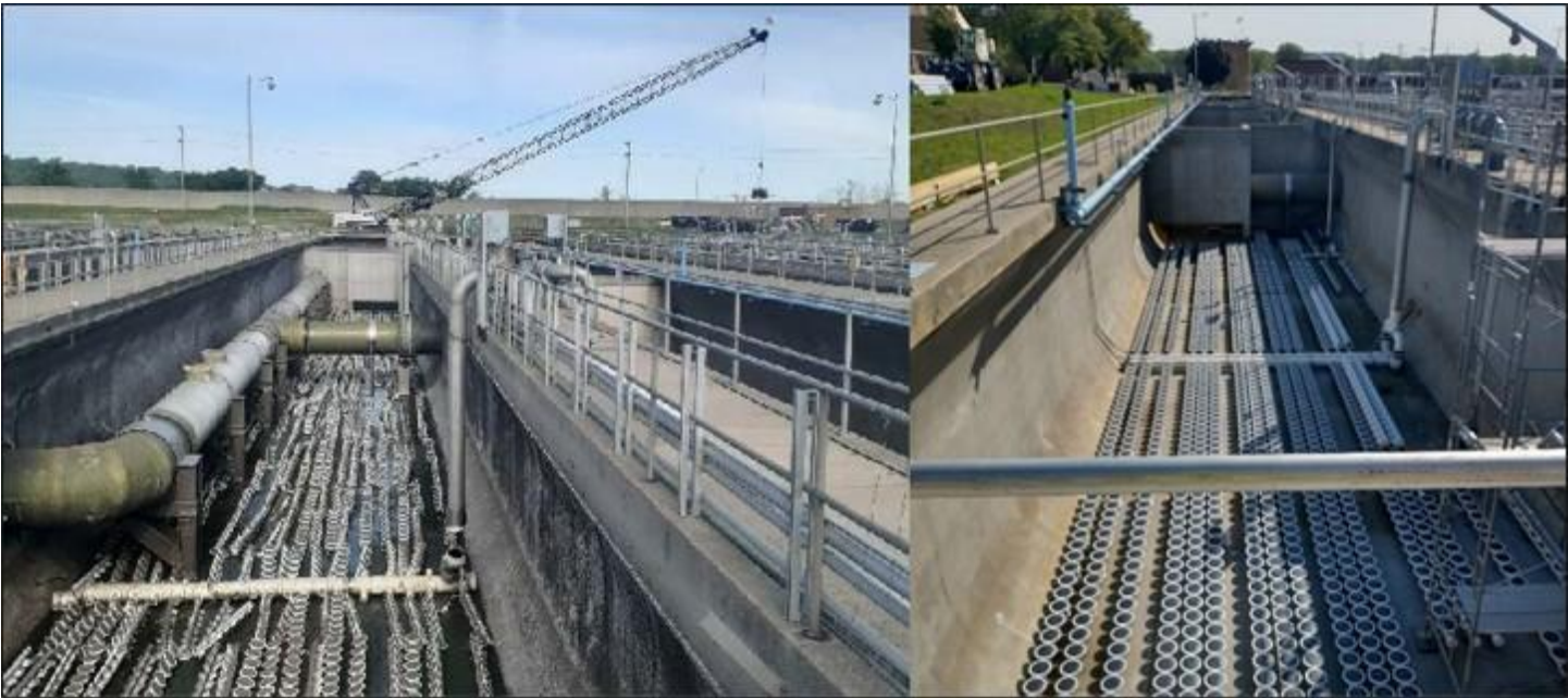
Left: Demolition of diffusers - Metro Facility’s secondary treatment. Right: Installation of diffusers - Metro Facility’s secondary treatment.
