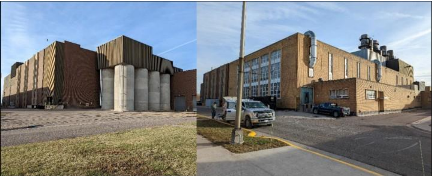
Left: 408 Building looking west.
