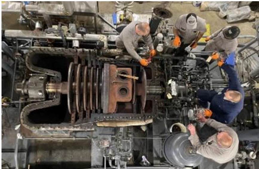
Metro Facility staff performing maintenance on the G7 steam turbine generator
