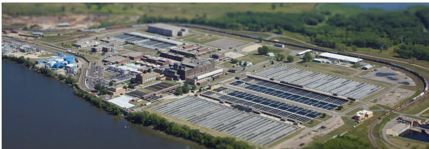
Metropolitan Water Resource Recovery Facility (WRRF)
