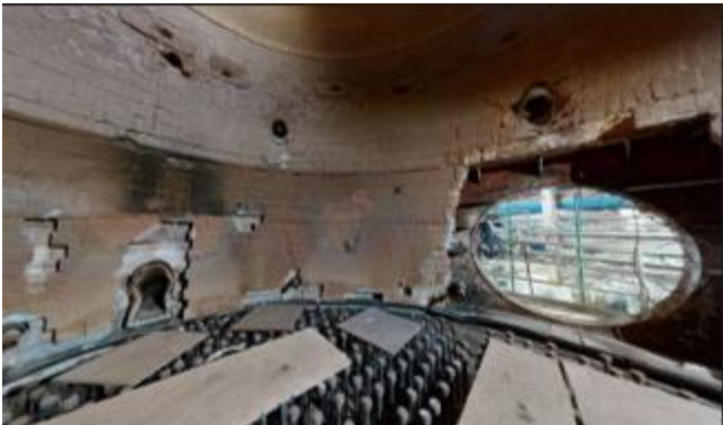
Incinerator Refractory Rehabilitation
