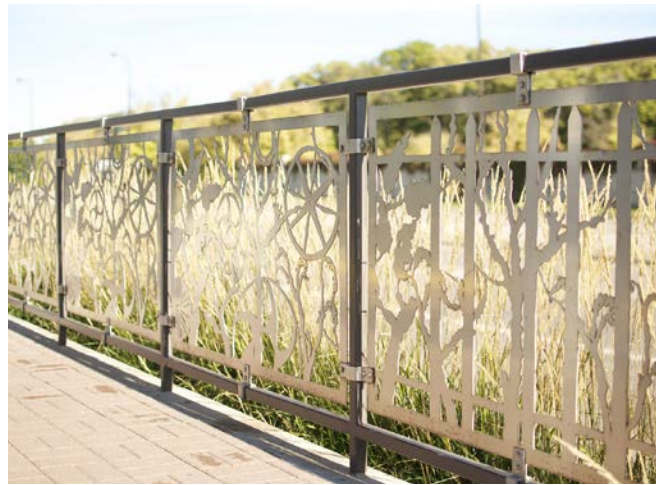
Railing Infill - Blue Line Metro Transit
